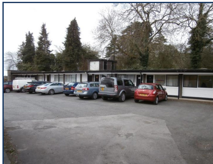
The photo above shows the self contained offices
